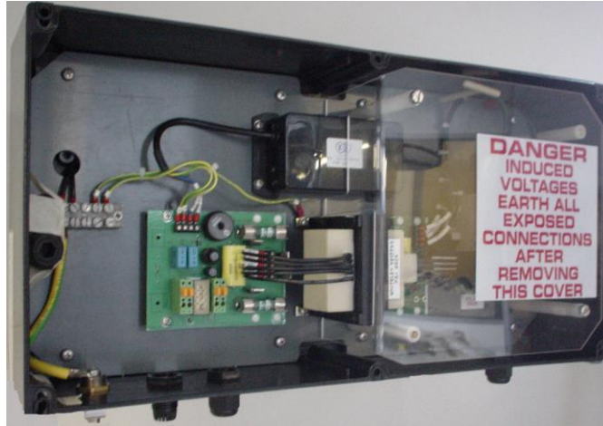
Internal View of Isolation Unit
