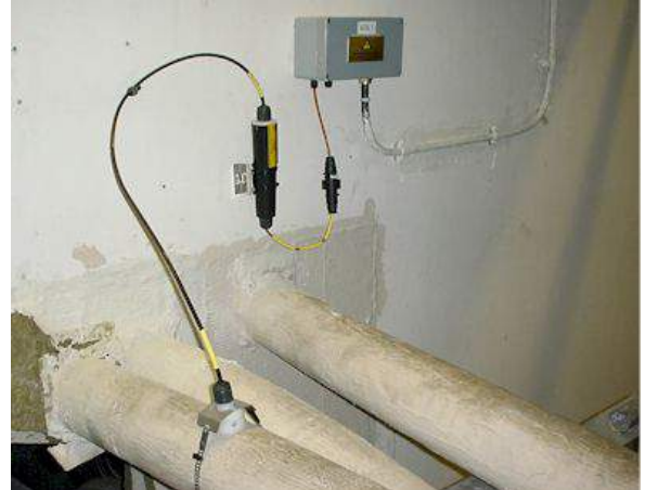
View of Sheath Temperature Sensor
